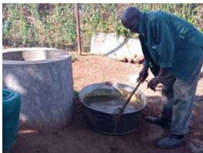
Mixing cow dung with water for feeding the digester
