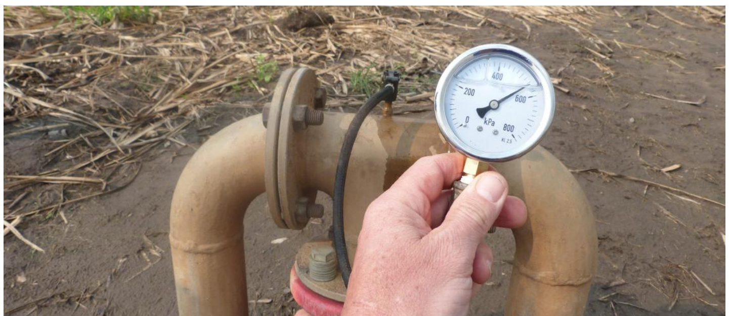
Figure 3: Measuring the pressure downstream of a hydrant
