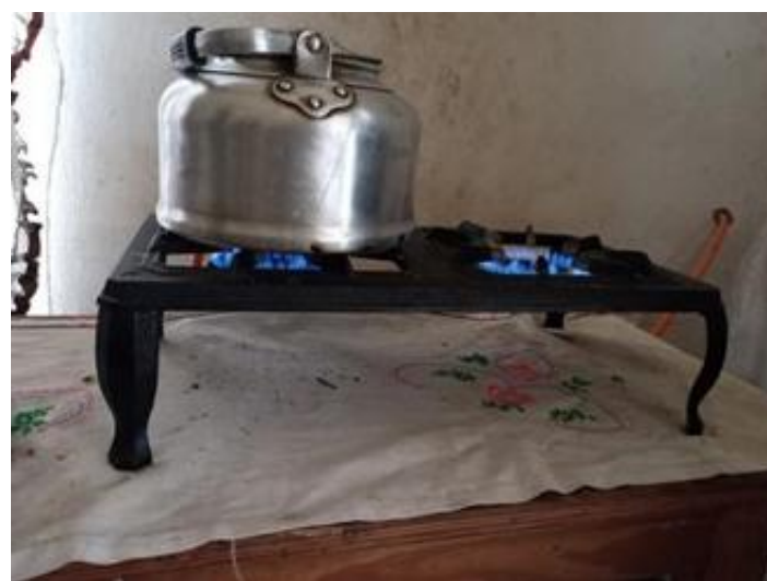
Operational gas stove. Status at 18 months post installation, indicating well fed biogas digester with good pressure.
