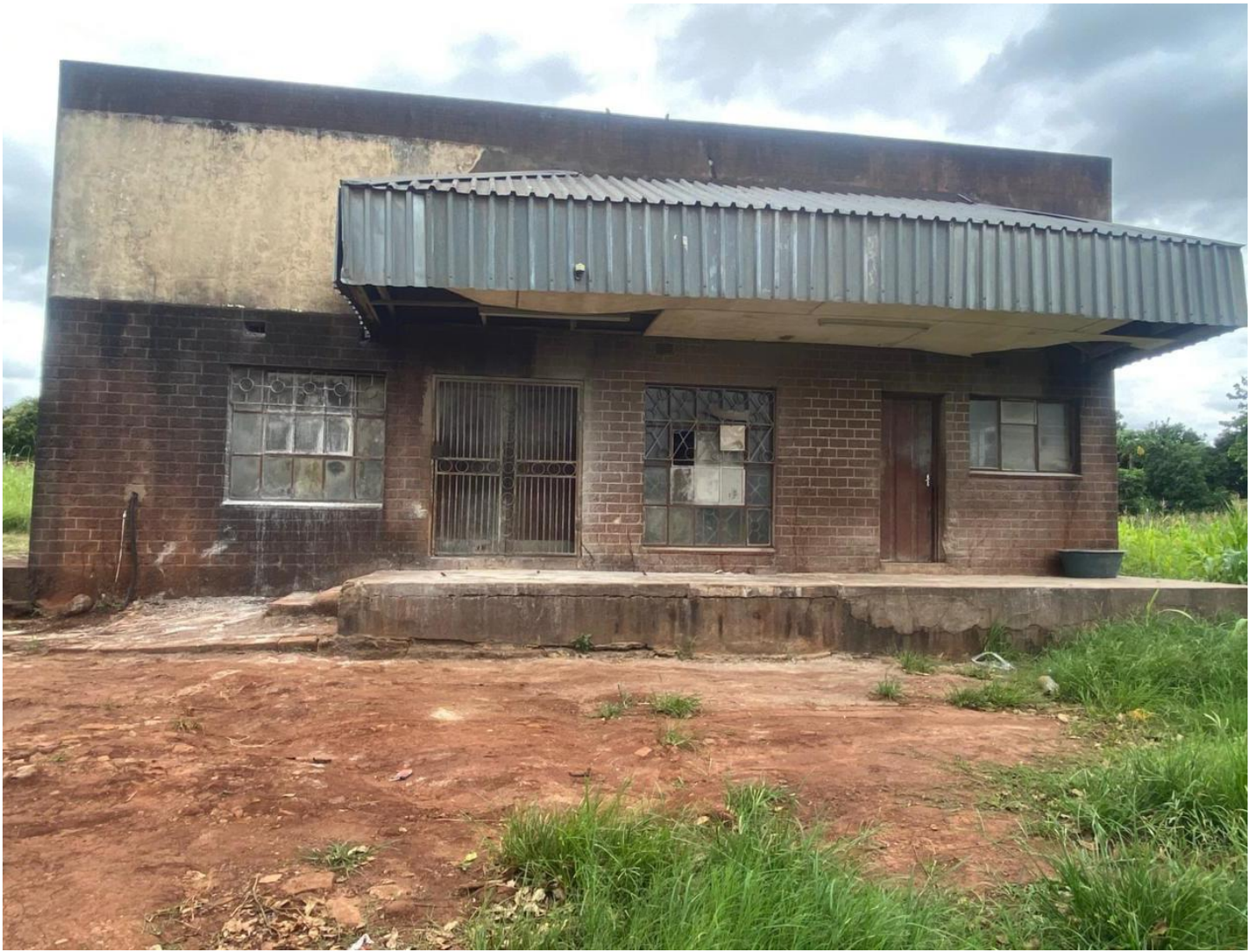
Figure 1: A maize milling facility in a rural village in the Vhembe District
