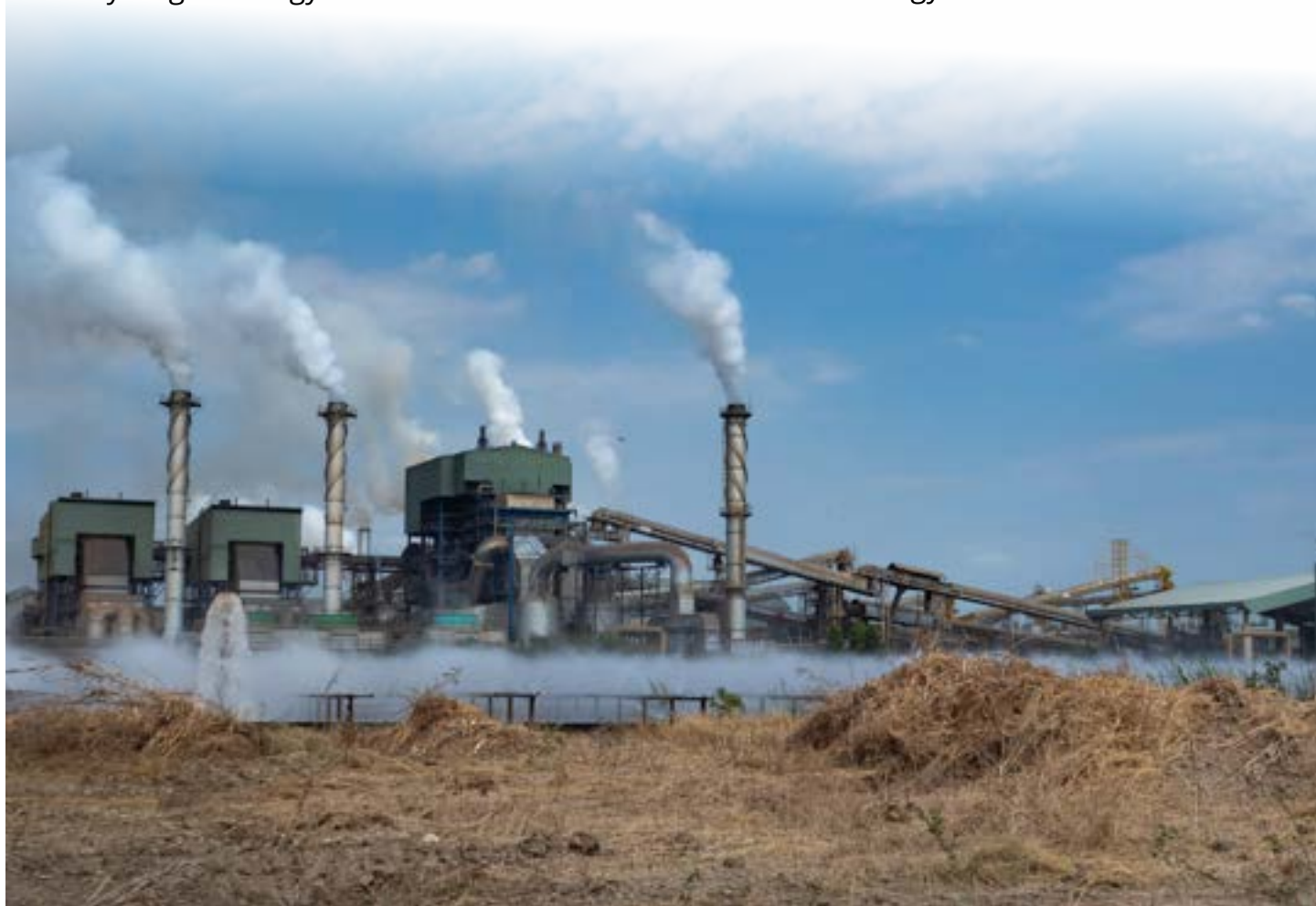
Figure 1 A sugarcane milling facility (Source: Vecteezy)
